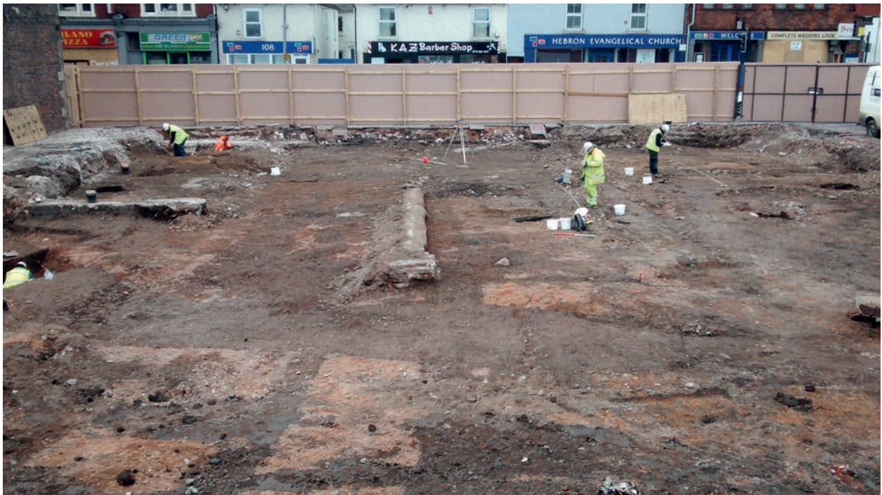
Figure 1.3 Area C (shot faces southwest).
