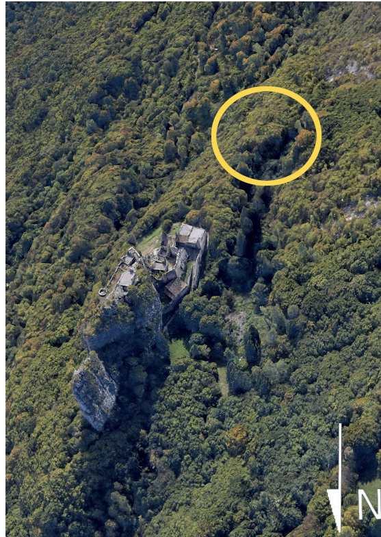
Figure 2: Panoramic view of Castel Corno and localization of the caves. (Image taken from Google Earth Pro V. 7.3.4.8642, on 31 August 2021).
