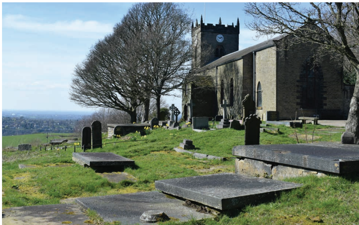
Figure 1.6. St. Thomas's Church, looking west, with Marple Ridge in the middle distance (left) and the Cheshire Plain beyond. Photograph by Graham Eyre-Morgan.
