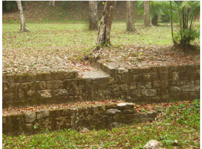
b) Photo of canal at the western embankment of Calzada Blom
