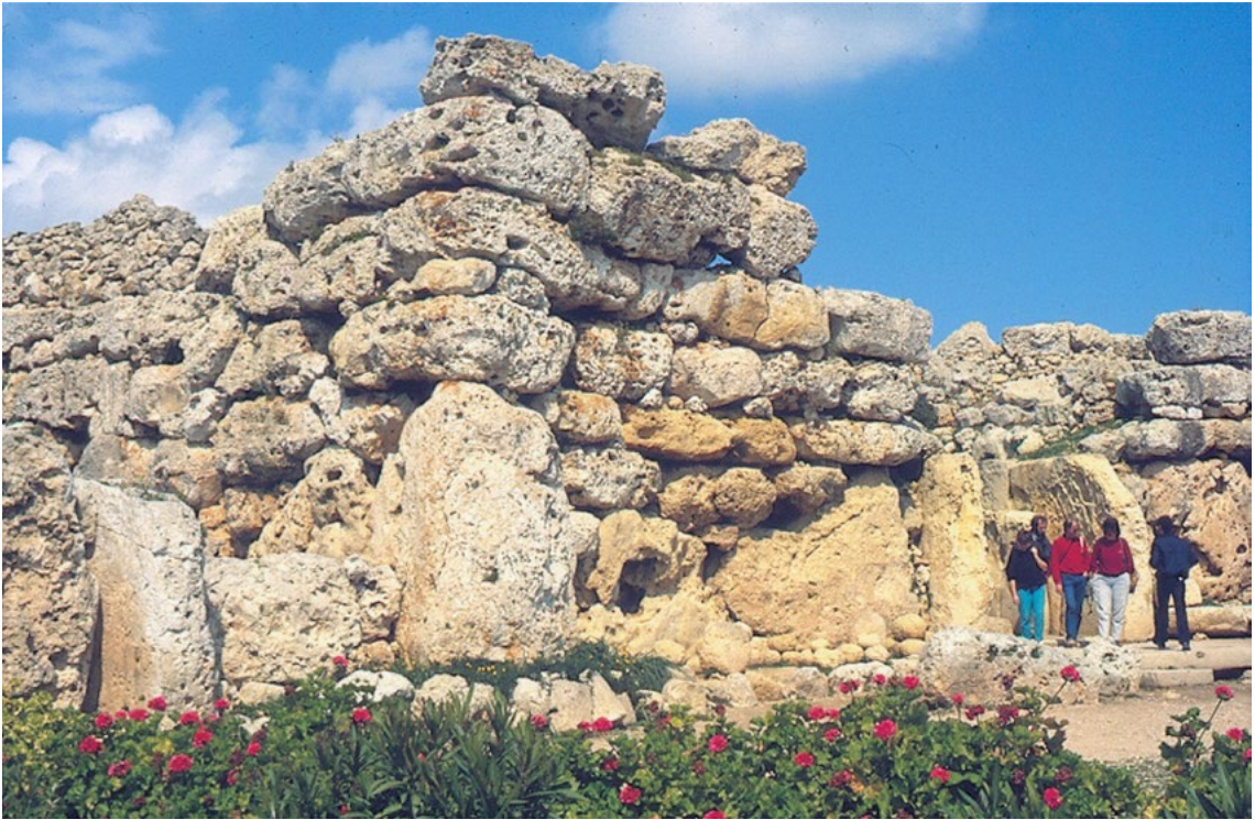
Figure 3: The impressive and exceptionally well-preserved façade of the south temple unit of Ġgantija, Gozo. The outer walls are built of blocks of the harder Coralline limestone. The walls flanking the entrance are in the softer Globigerina limestone.
