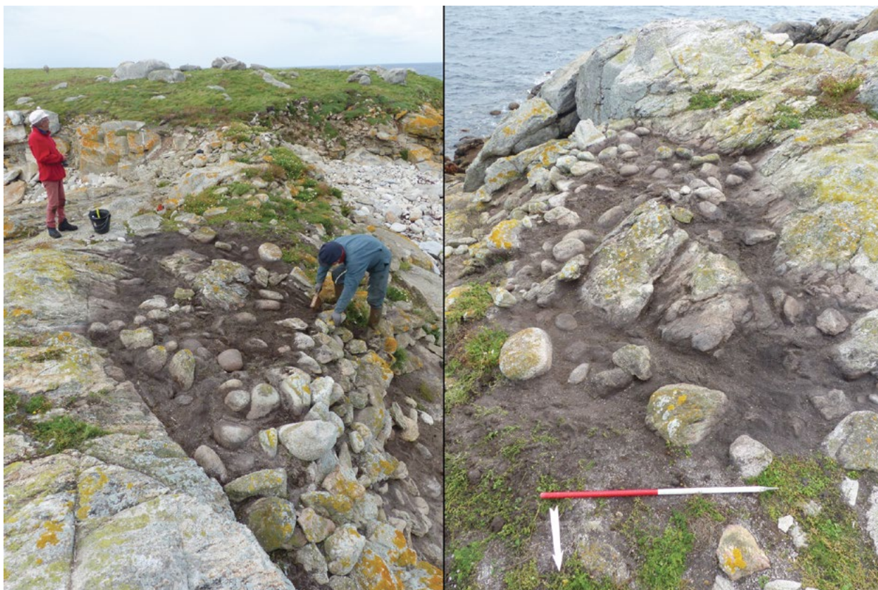
Figure 8: Cleaning the southern extremity of the rampart. View from the south side being cleaned and view from the north after cleaning (photographs H. Duval).
