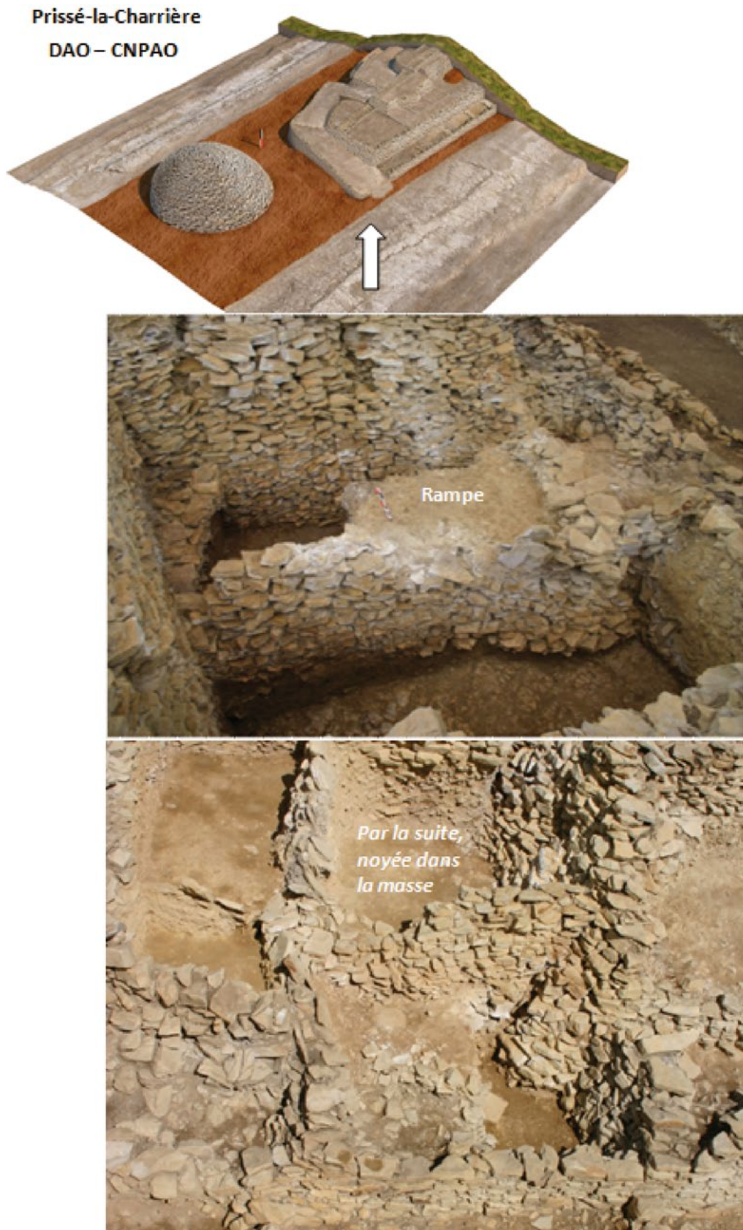
Figure 13: Technical structures embedded in the mass, following a pre-established plan and perfectly stable during the whole duration of construction. Prissé-la-Charrière – Photo. L. Laporte.
