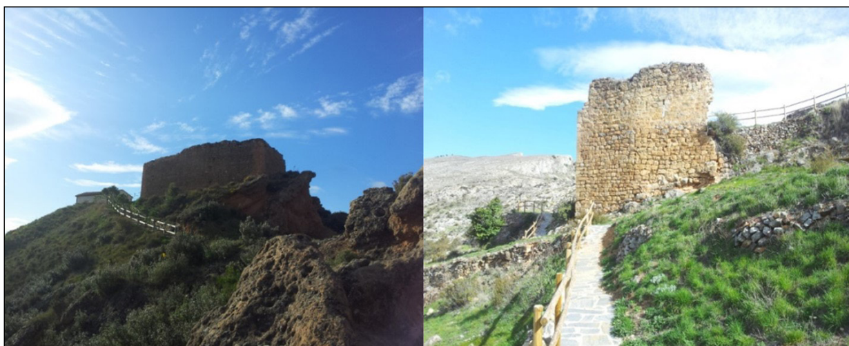
Figure 11. Left: Tower of Herce; right: Torre of Muro de Aguas (author).
