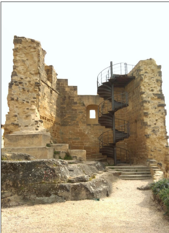
Figure 4. Stairs in Briones (author).
