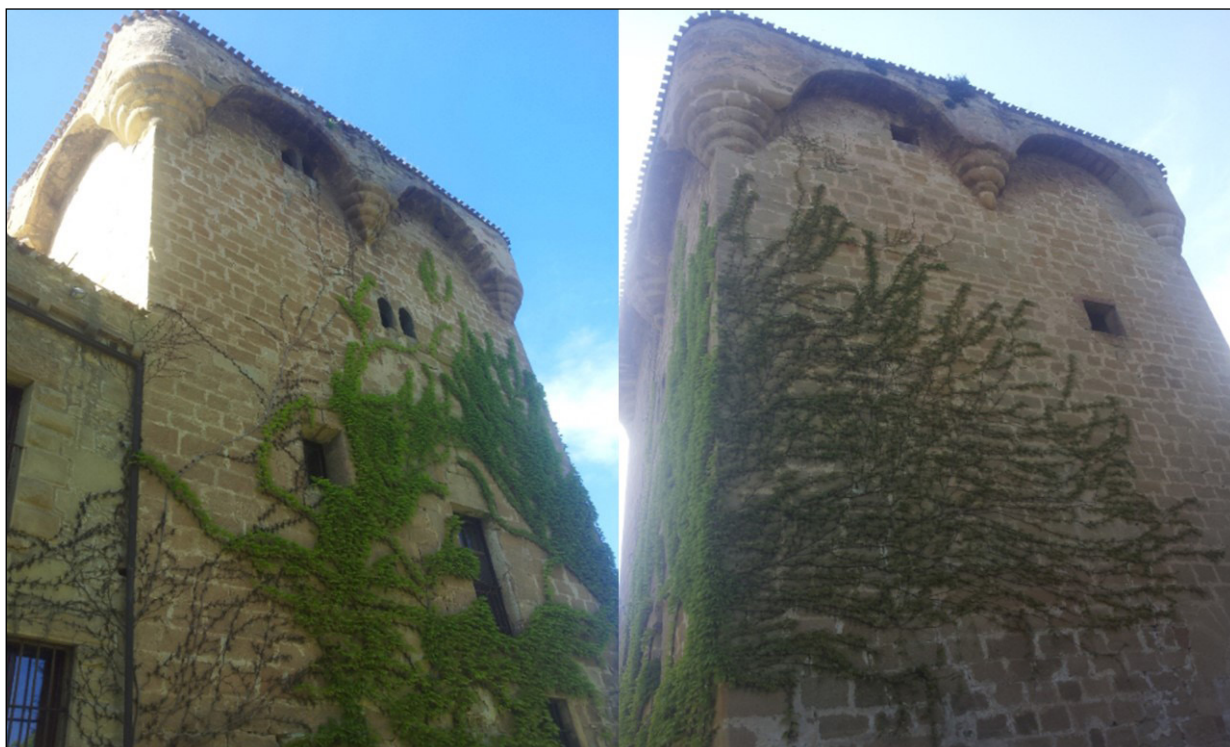
Figure 10. Tower of Torremontalbo (author).
