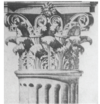
Figure 131. A reconstruction of a Corinthian capital from the Temple of Castor and Pollux (Gütschow)
