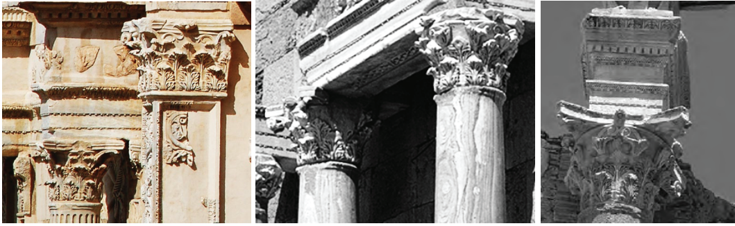
Figures 237A-B. A Corinthian capital and a pilaster from the Arch of Septimius Severus (Researchgate)*
