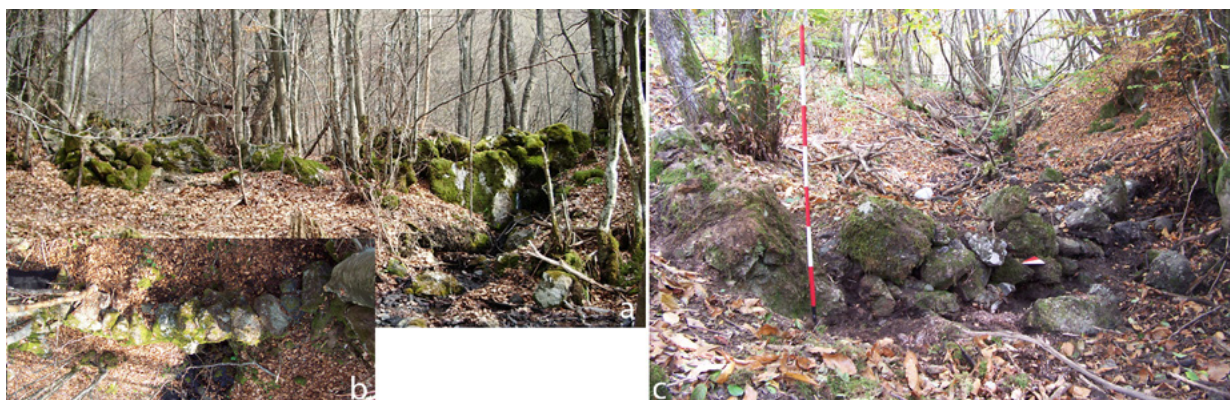
Figure 4.9. Filtering walls of the Lungaie (a) and Moglia del Chirlo (b) wetlands (from Montanari & Stagno 2015, Figure 3).
