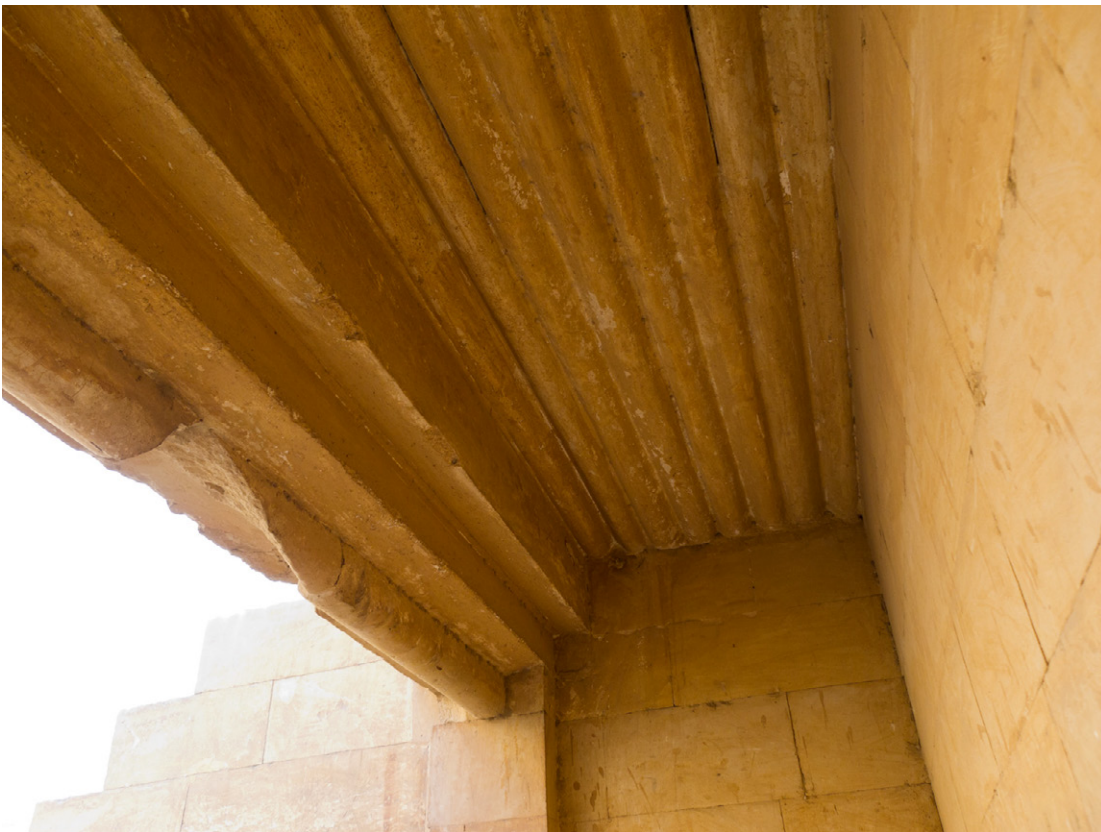
Figure 1. Imitation of wooden beams sculpted on the ceiling, Temple T, Saqqara. (© Kairoinfo4u, Flickr).
