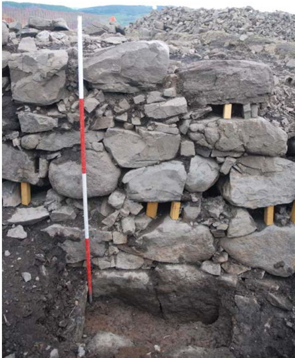
Figure 3.69: Detail of the internal face of Wall E in Trench A, showing bedrock at the base, and sockets for transversal timbers.
