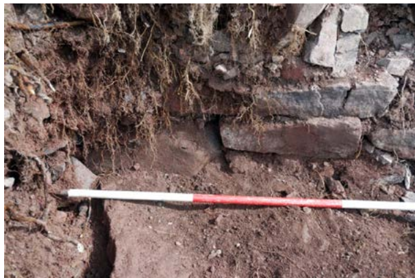
Figure 6.25: Detail of the join of the transverse and inner walls shown in Figure 6.24.
