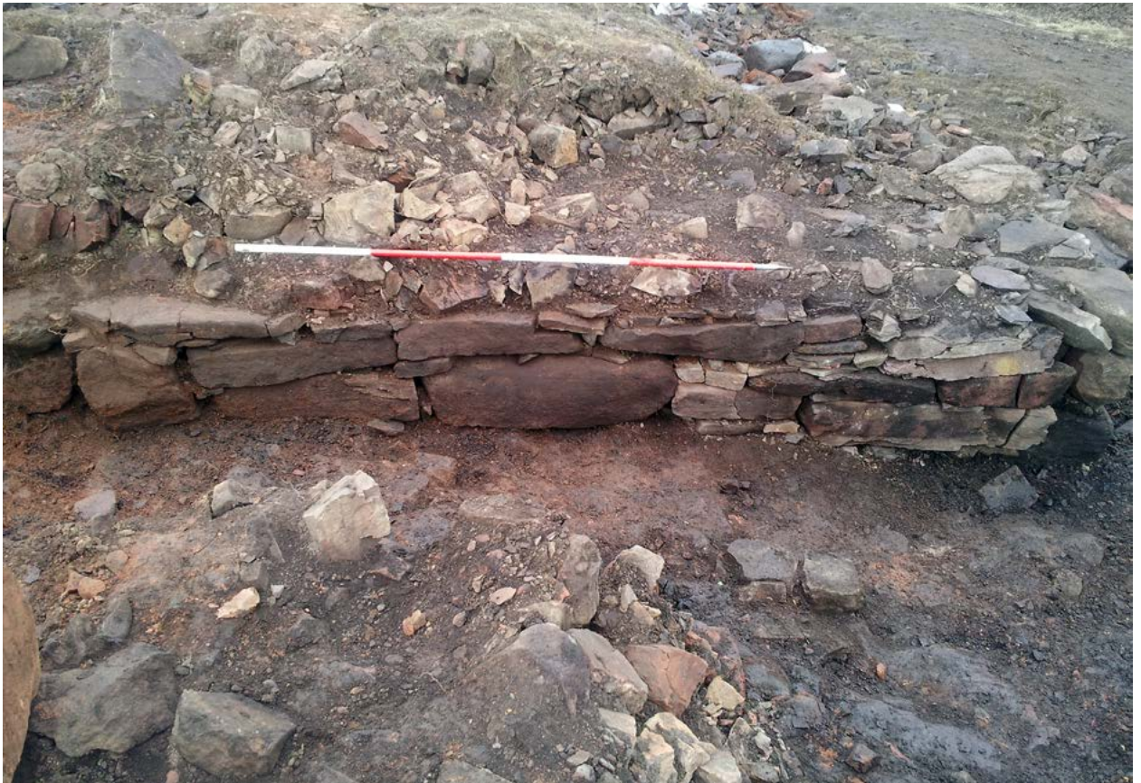
Figure 3.26: The north-facing façade of the entrance passage [C008/2016] detailing the use of both Old Red Sandstone and local stone built, with the wall constructed directly onto the bedrock.
