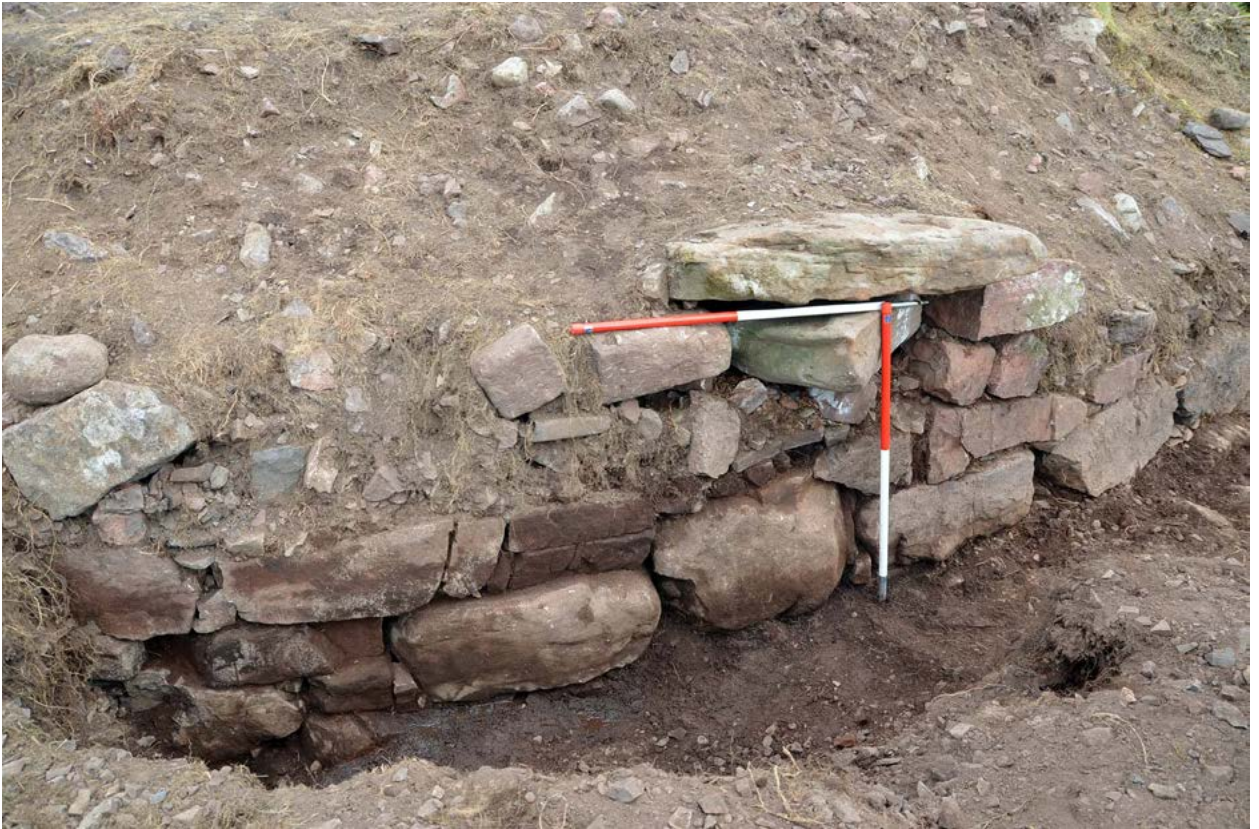
Figure 6.11: The external façade of the inner wall in 2017, constructed onto the bedrock. The extent of erosion is clear through comparison with Figure 6.4.
