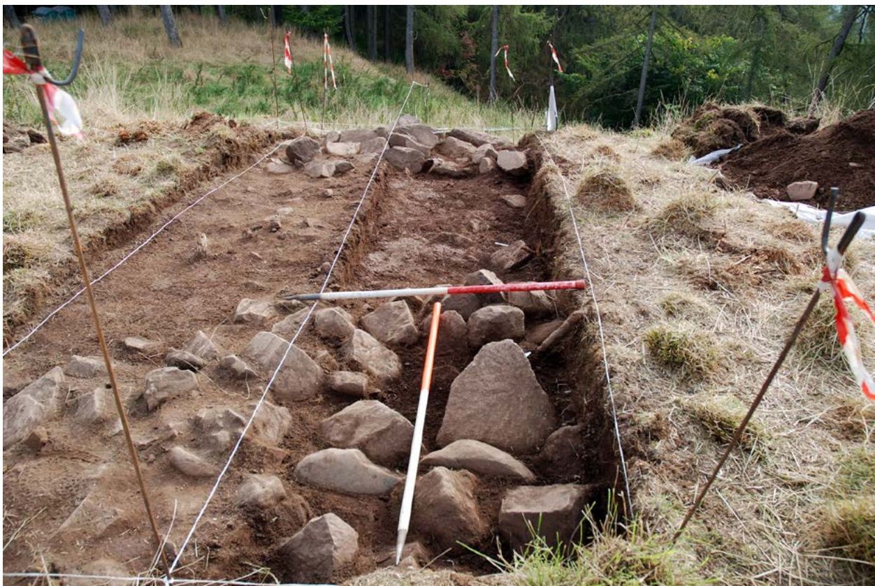
Figure 2.12: Working shot of Rampart A [210] showing the inner stone facing [209] in the foreground with the outer stone facing [203] beyond.
