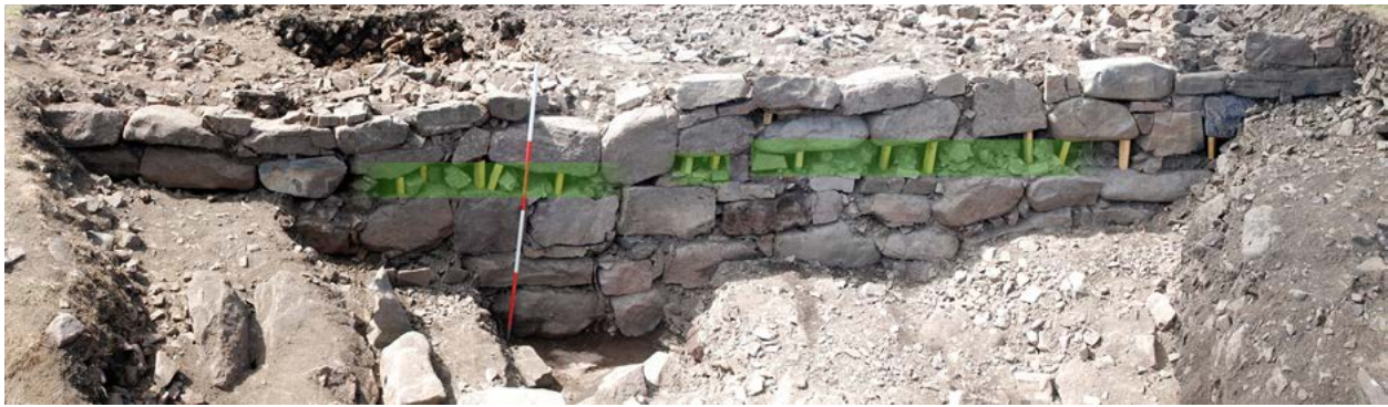
Figure 3.95: Photo montage of the external face of Wall E.
