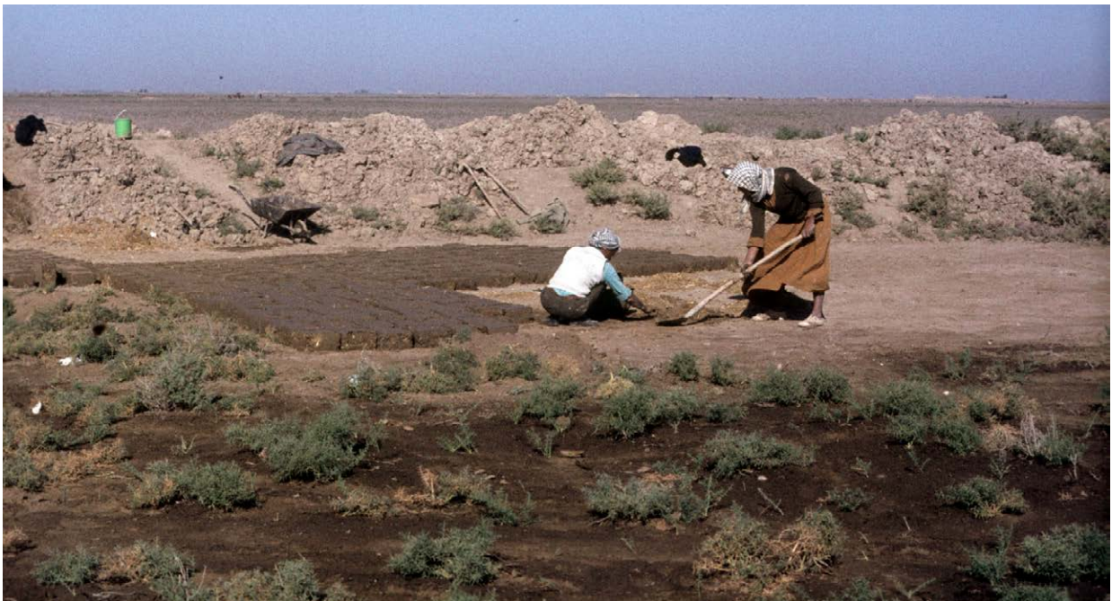
Figure 3.7. Making mud-bricks for the excavation house, down by the canal. September 1976.
