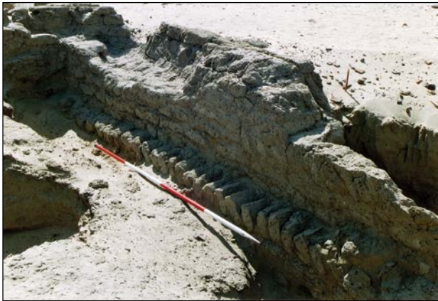
Plate 4.8. Building B12. Foundation course of the south wall visible in Room XVIII, looking south east – scale bar 2m.
