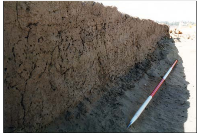
Plate 4.34. Building B5. Mud render on the external face of the north wall, looking west – scale bar 2m.
