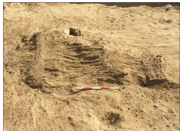
Plate 6.10. Building F1, Room IX. Articulated roof timbers – scale bar 500mm.
