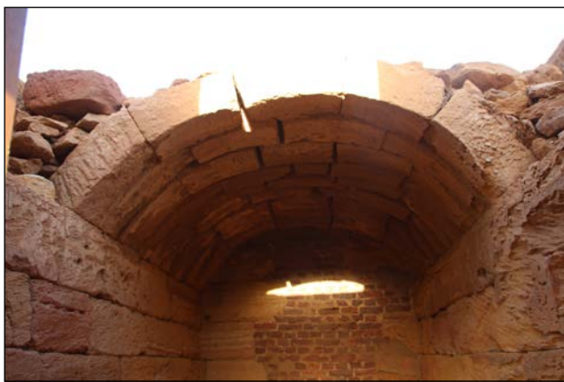
Plate 12.14. The segmental vault roofing the offering chapel of Pyramid Beg.N.6. in the North Cemetery at Meroe.
