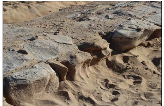
Plate 16.26. The heavily eroded face of the south wall.
