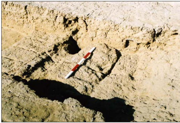
Plate 10.3. Building Z1, Room II. The threshold, 'pivot' and sockets for the wooden elements of the steps looking south west – scale bar 500mm.
