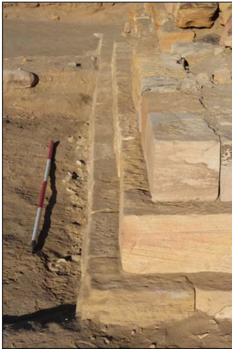
Plate 11.133. Grid square (JC3). Grave 12 – the south face of the pyramid and the construction trench filled with small stones, looking west.
