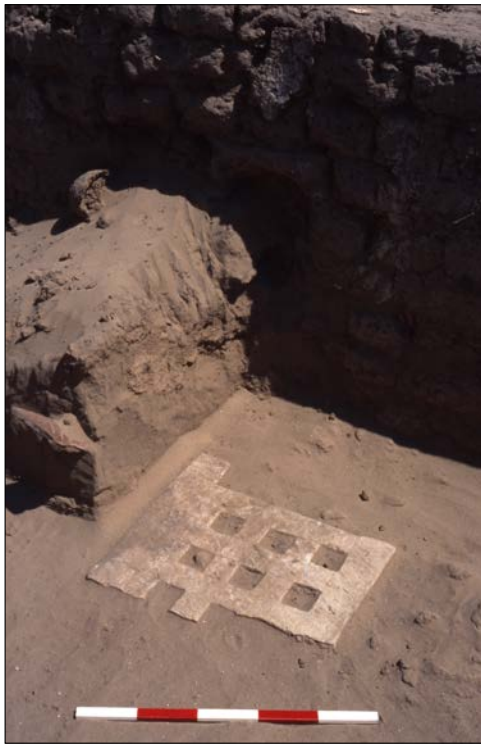
Plate 3.32. Building A1, Room IV, surface(AB5)58/245 with a white sandstone window grille set into it – scale bar 500mm.
