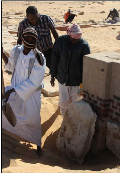
Plate 16.23. Placing a large stone slab, which was subsequently covered with sand level with the ground surface, to protect a fine cartouche of Tabarqa.
