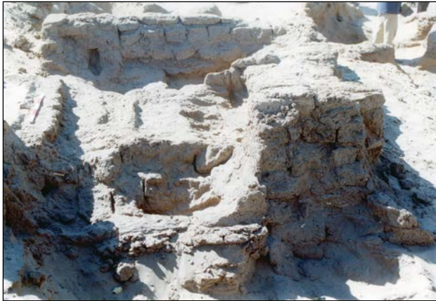
Plate 4.32. Building B14, Room XXVI, looking south. The external doorway is on the left, the primary surface with the impressions of the timber threshold and the socket for the sill in the south wall can be clearly seen. The masonry to the right is the extension of the vestibule and the later mud-brick threshold.
