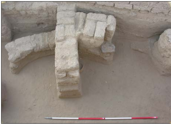
Plate 3.14. Building A3. Doorway through south wall of the building after removal of contemporary floor levels. The pivot stone remains in situ. The wall at 90° is part of Building A4 – scale bar 2m.
