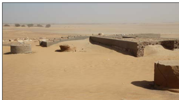
Plate 16.21. Build-up of wind-blown sand in the north-east corner of the First Court.
