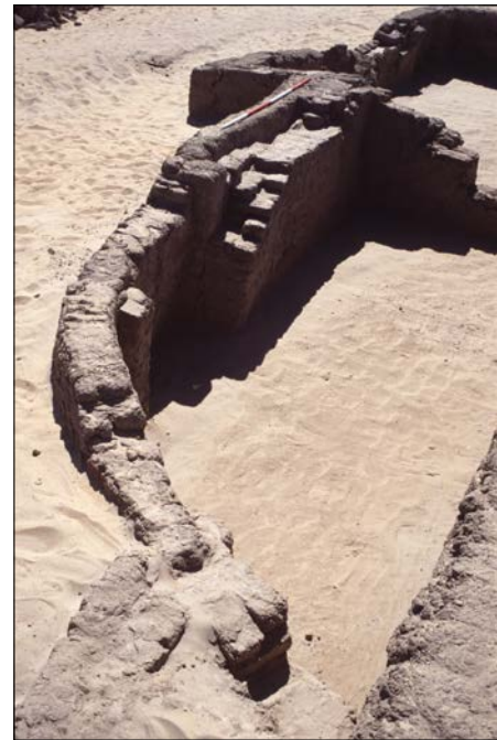
Plate 3.11. Building A3. The highest surviving section of wall with the Phase II buttress inserted against the inner face of the east wall – scale bar 2m.
