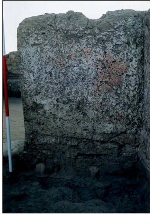
Plate 3.25. Traces of wall paintings on the east wall of Room A1-III to the south of the doorway – scale bar 1m.
