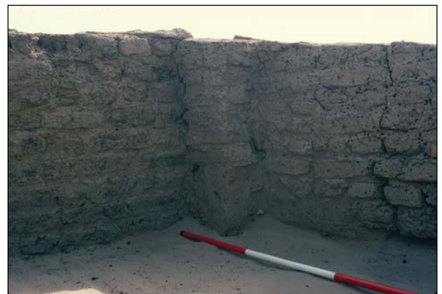
Plate 4.61. Building B1, Period 2, Phase 3 – The buttress in the south-east corner of Room II abutting the Phase 1 and 2 walls, looking south east – scale bar 1.5m.
