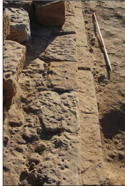
Plate 12.7. Setting-out lines on the south face of Pyramid S5.
