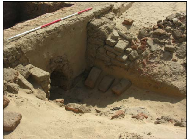
Plate 7.33. Building F3. The west stoke-hole the three mud bricks resting on ash deposit (FT3)62 and the south revetting wall, looking south east – scale bar 2m.
