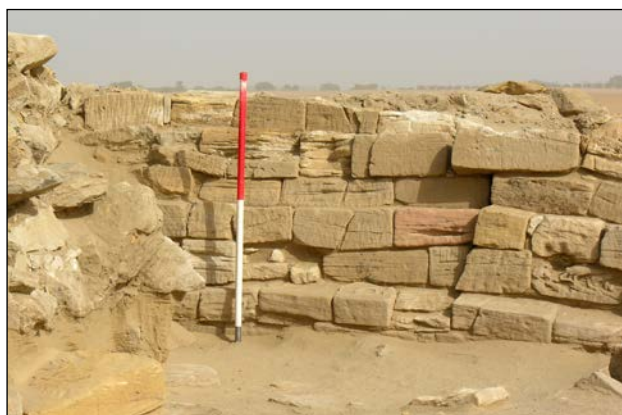
Plate 12.9 The central part of the south face of Pyramid S2 with the rubble of its collapse on the left.
