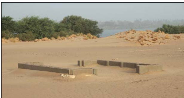
Plate 16.32. The Western Kiosk after the preservation work, looking north west.
