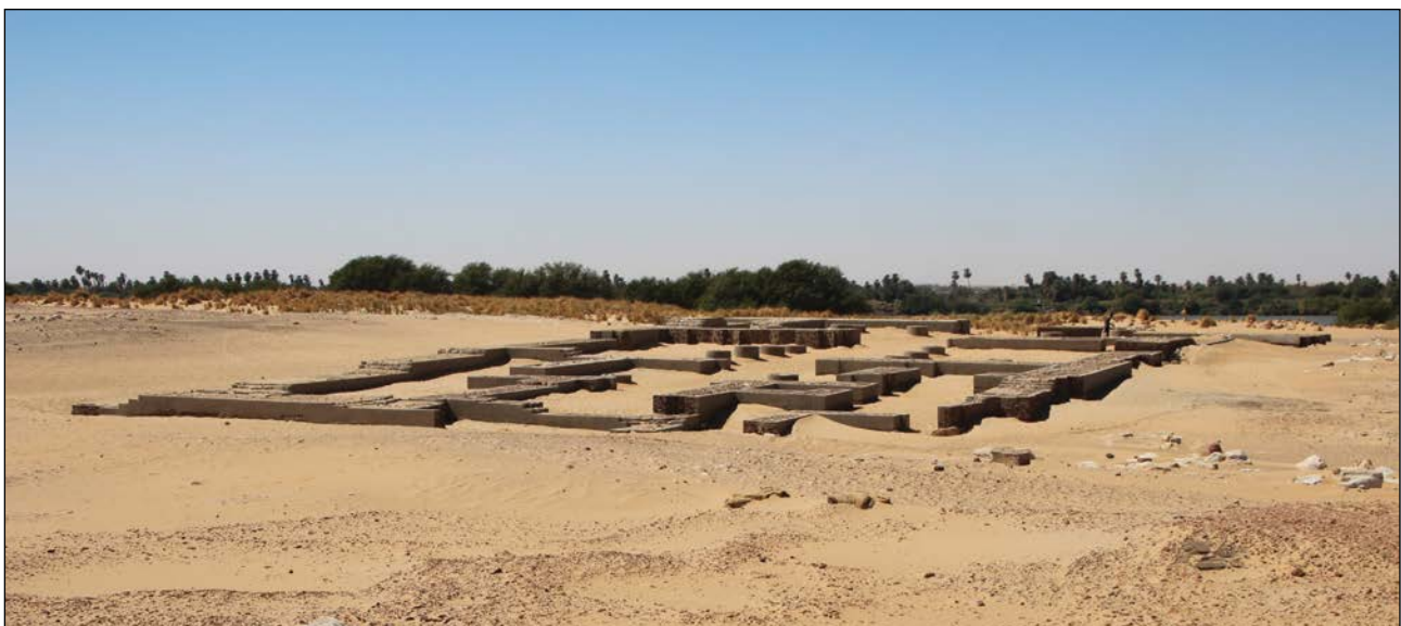
Plate 16.29. Temple T after the preservation measures, looking west south west.
