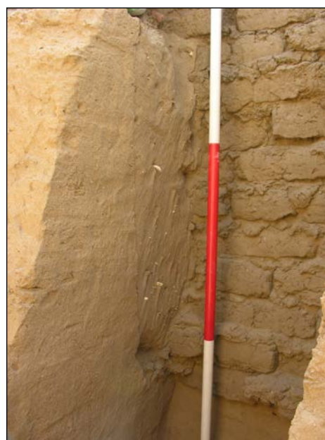
Plate 7.21. Building F3. The north edge of the construction pit and the north wall – scale bar 1.5m.
