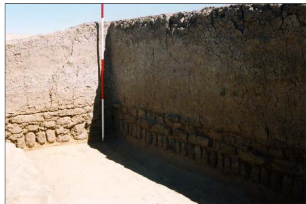
Plate 10.2. Building Z1. The north and east walls of Room I showing foundations and mud mortar render above the primary floor level looking north east – scale bar 2m.
