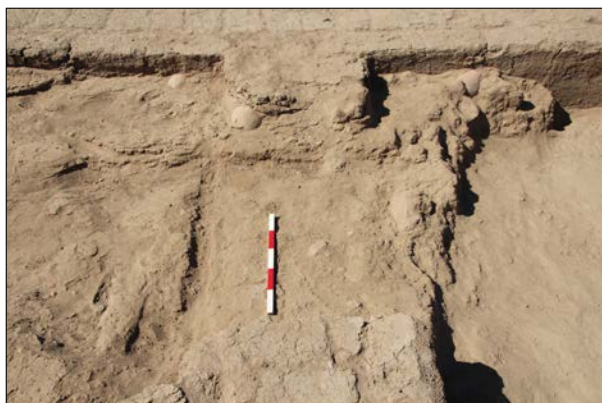
Plate 6.20. Building F1, Rooms II-III. The reinstated doorway, looking west – scale bar 500mm.
