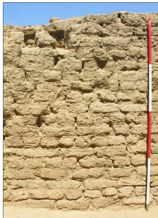
Plate 3.42. Building A2: the windows in the north wall of Room A2-VII – scale bar 2m.
