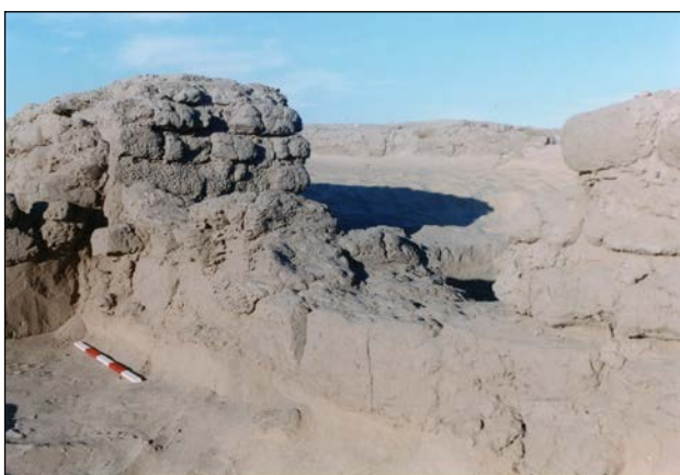
Plate 4.37. Building B5. Foundations of the wall between B5-X/XII and B5-VIII/XIV on its western face, looking north east – scale bar 500mm.
