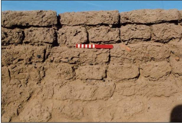
Plate 4.7. Building B12. Detail of the brickwork – scale bar 200mm.
