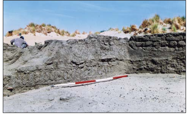
Plate 4.9. Building B12. The west wall of Room XVIII, looking north west – scale bar 2m.
