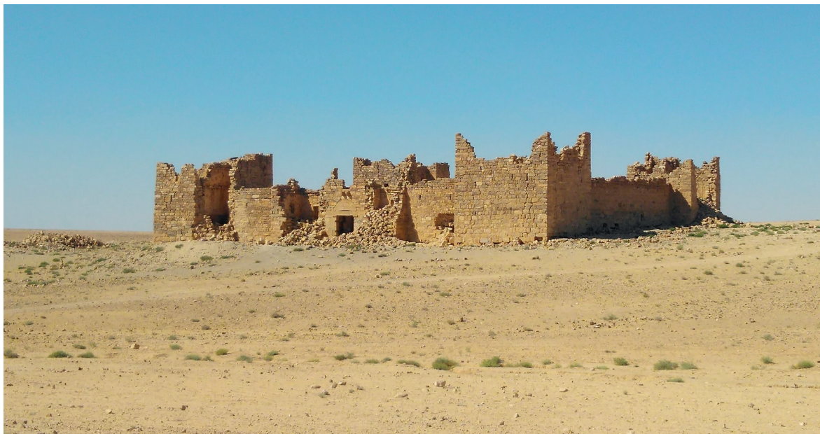
41. Qasr Bshir (Jordan) is typical of the forts in the desert, yet unique in its state of survival
