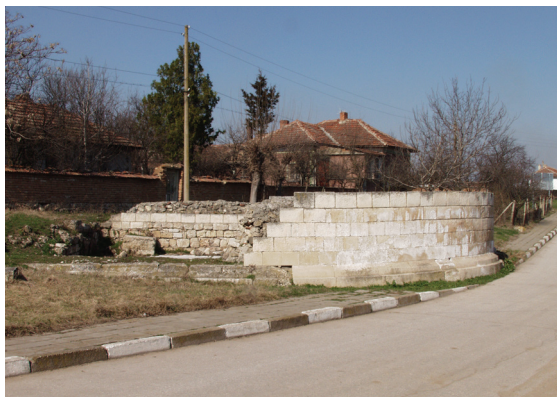
80. A partially reconstructed bastion in the village of Gigen (Oescus)
