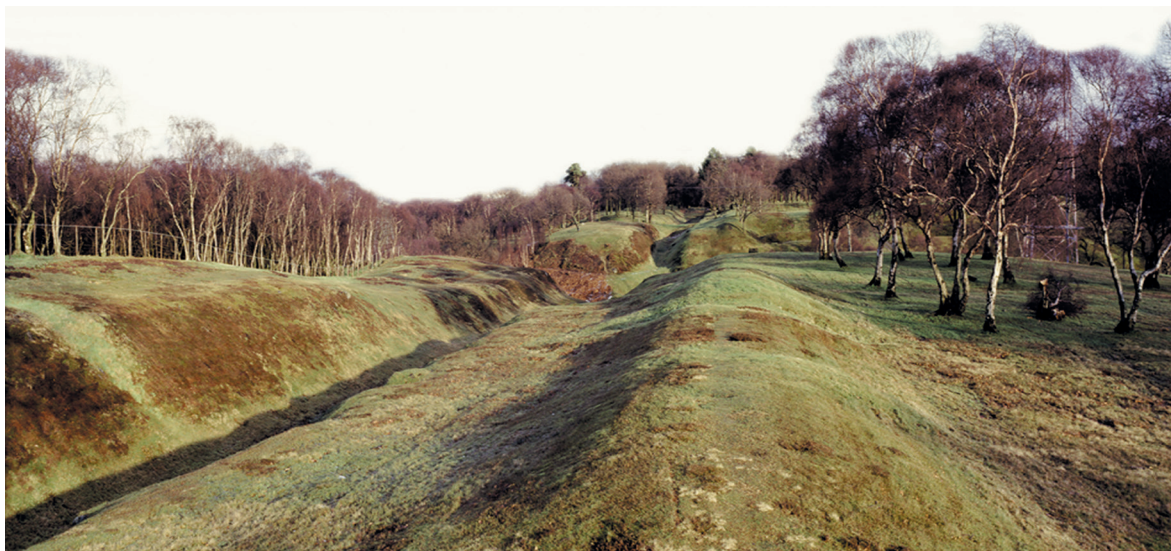
43. The Antonine Wall (Scotland, UK) was built of turf, which survives as a low mound; the ditch is to its left Стената на Анонинус (Шотландия, Великобритания) изградена от торф
