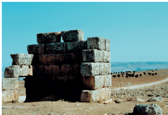
30. Towers, such as this one in Turkey, aided communication along the frontier roads
