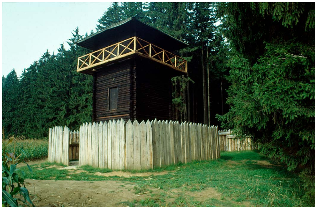
Figure 50. The timber tower at Mahdholz recently created, one of the many treats provided by the Denkmalpflege in Baden-Württemberg
