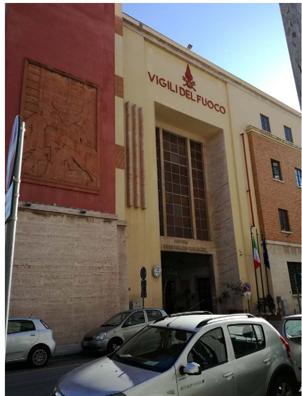
Figure 5.1: Entrance to the fire station at the Via Scarlatti, Palermo (source: author).
