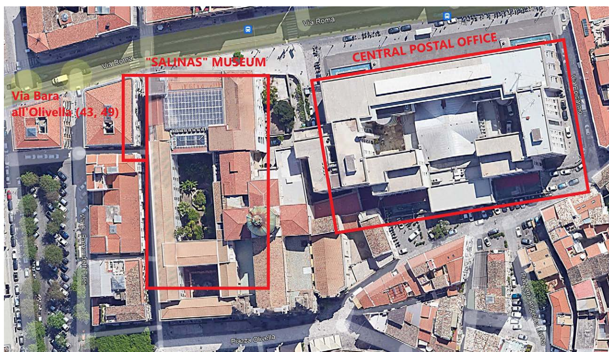
Figure 5.6: Satellite view of 43 and 49 Via Bara all'Olivella, the 'Salinas' Museum, and the central post office (source: Google Earth).
