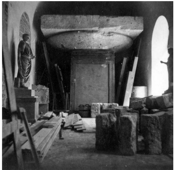
PAL.26.71 | AMARAS | pictures | 1 side | 1943 | inv. no. 8292 | 13x18 | Palermo, National Museum: internal section of the cloister arranged for the anti-aircraft protection (courtesy of Museo Archeologico Regionale 'A. Salinas').
