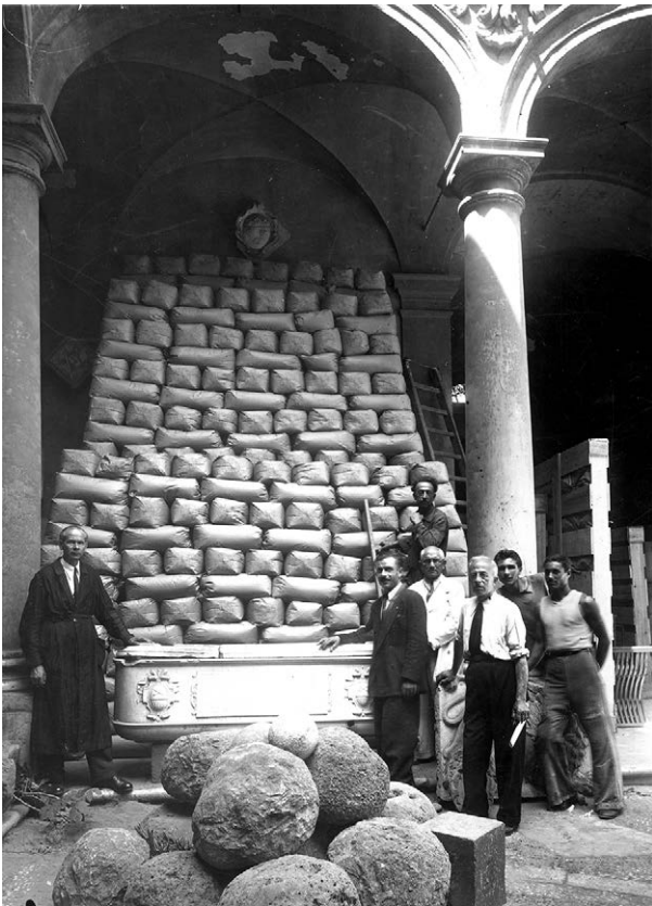
PAL.26.61 | AMARAS | pictures | 1 side | 1943 | inv. no. 2209 | 13x18 | Palermo, National Museum: workers and custodians installing protective sandbags in the cloister (courtesy of Museo Archeologico Regionale 'A. Salinas').
