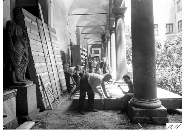
PAL.26.66 | AMARAS | pictures | 1 side | 1943 | inv. no. 7593 | 13x18 | Palermo, National Museum: workers and custodians preparing wooden box for the anti-aircraft protection (courtesy of Museo Archeologico Regionale 'A. Salinas').
