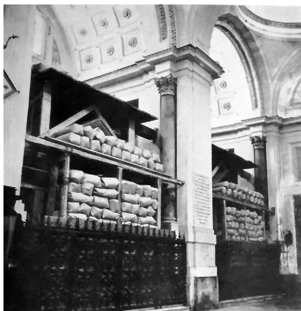
Figure 2.12: Scaffolding and sandbags protecting Palermo's Norman Cathedral (source: VV.AA. 1942b).
