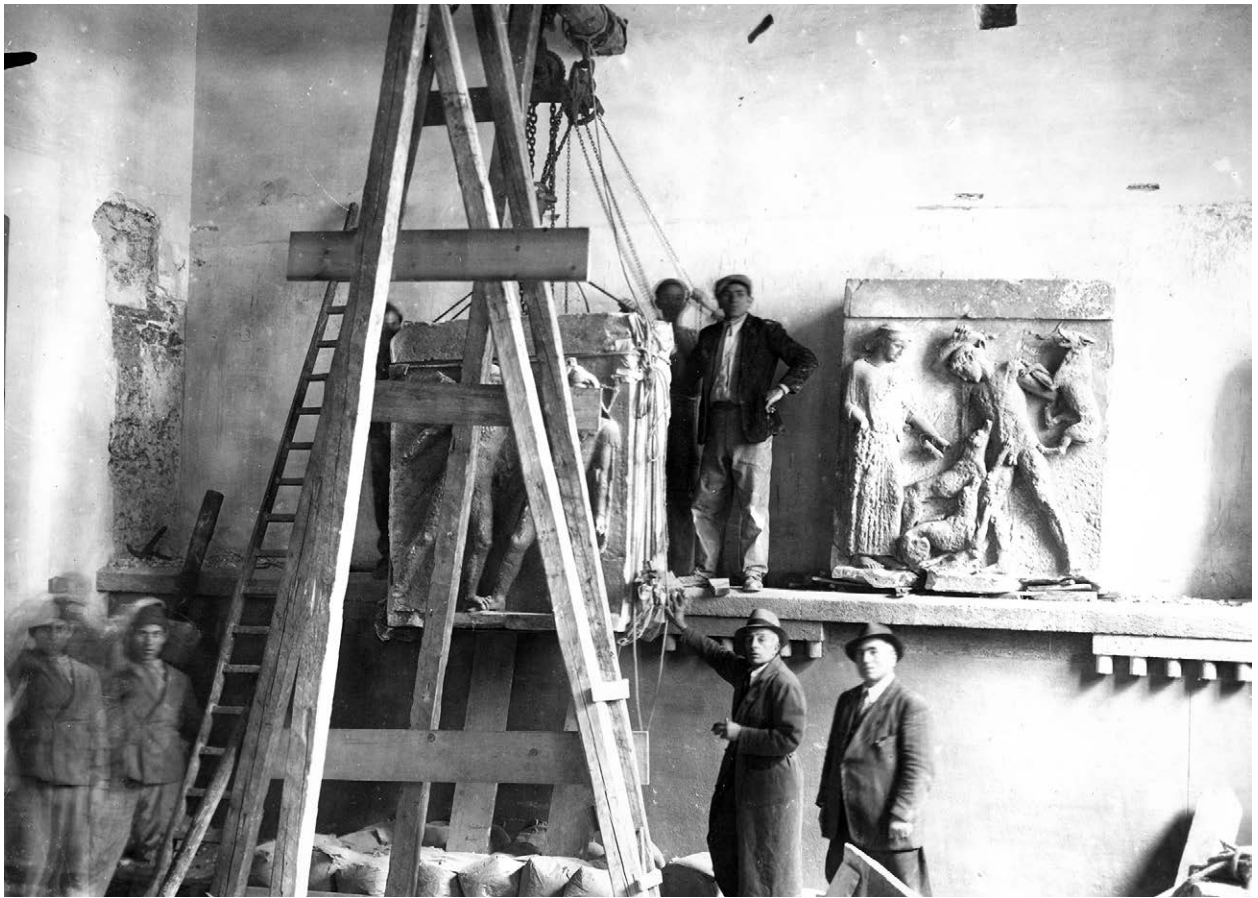
Figure 4.18: Workers installing protective scaffolding around the Selinunte metopes at the National Museum (courtesy of the Archaeological Museum 'A. Salinas', inv. no. 7598, PAL.26.68).
