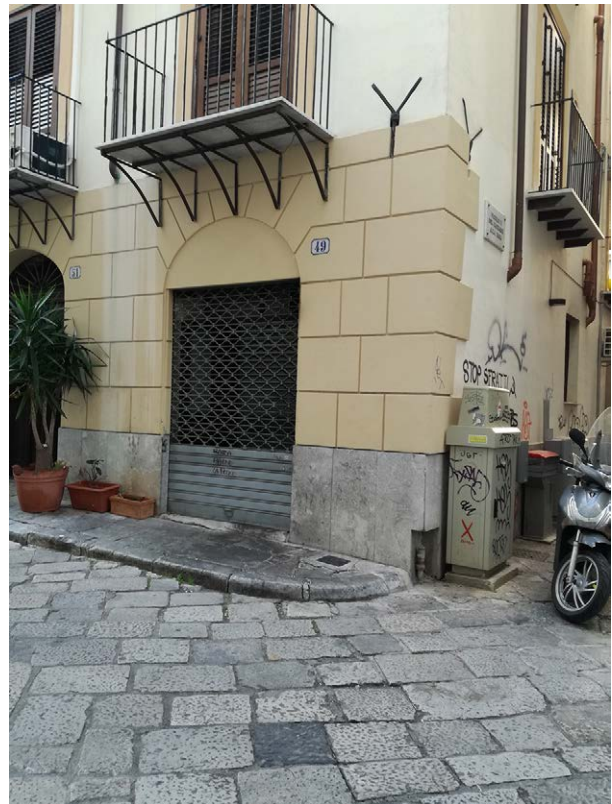
Figure 5.5: Entrance to 49 Via Bara all'Olivella (source: author).
