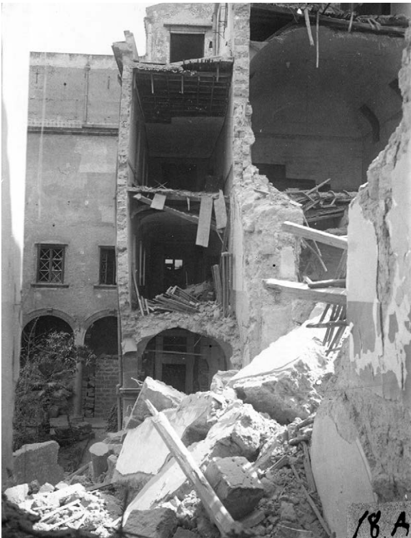
PAL.26.57 | AMARAS | pictures | 1 side | 1943 | inv. no. 8039 | 13x18 | Palermo, National Museum: view of damaged sections of the museum (courtesy of Museo Archeologico Regionale 'A. Salinas').
