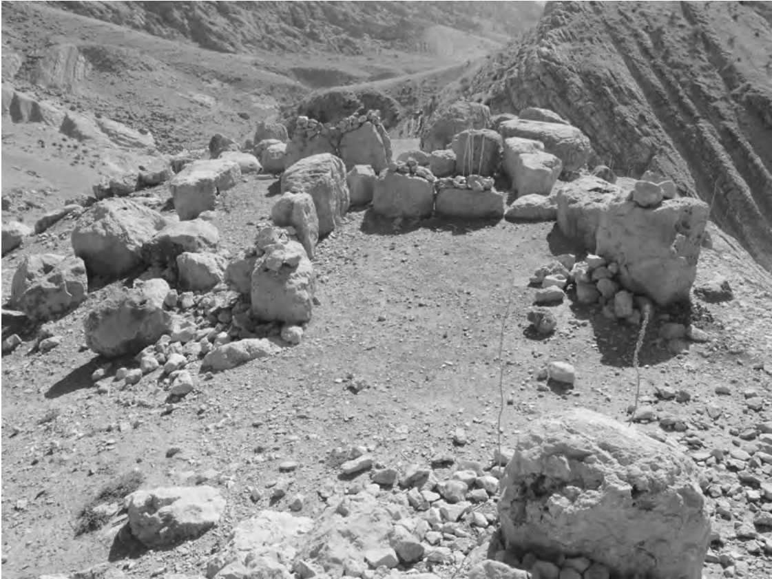
Figure 5.32 - Shami Valley, area of Saleh Vand: ruined building
