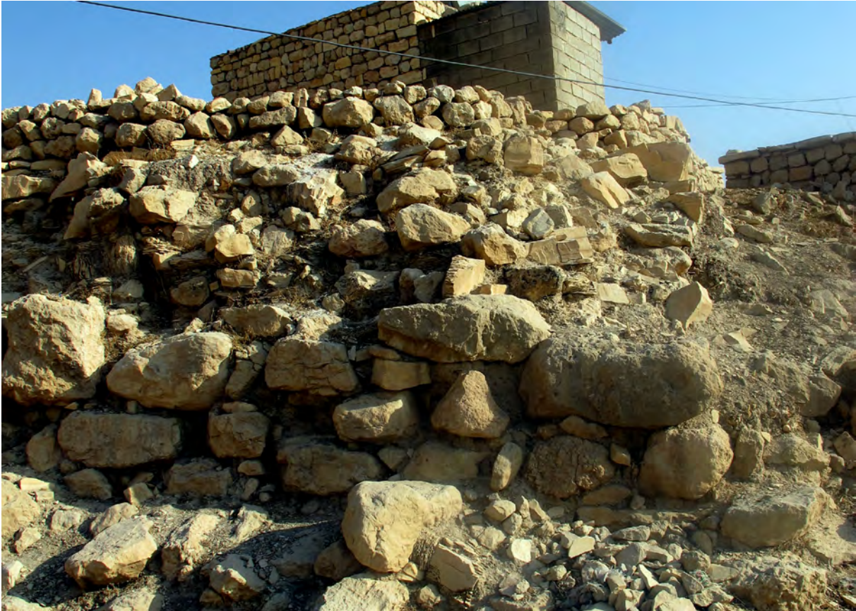
Figure 6.9 - Upper Terrace. South retaining wall. Detail of the southeast corner
