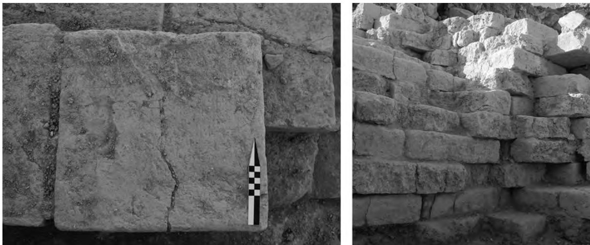
Figure 6.53 - Trench 3. Detail of a squared brick and brickwork seen from the hole in SU 1
