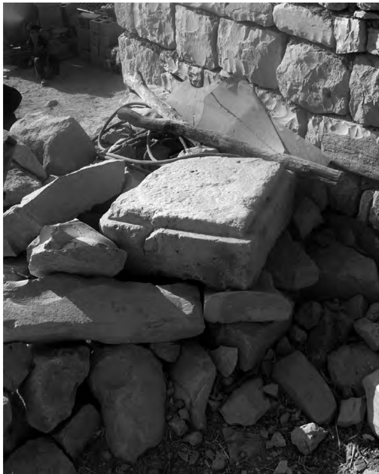
Figure 2.6 - Stone squared column base loose on surface of the Upper Terrace
