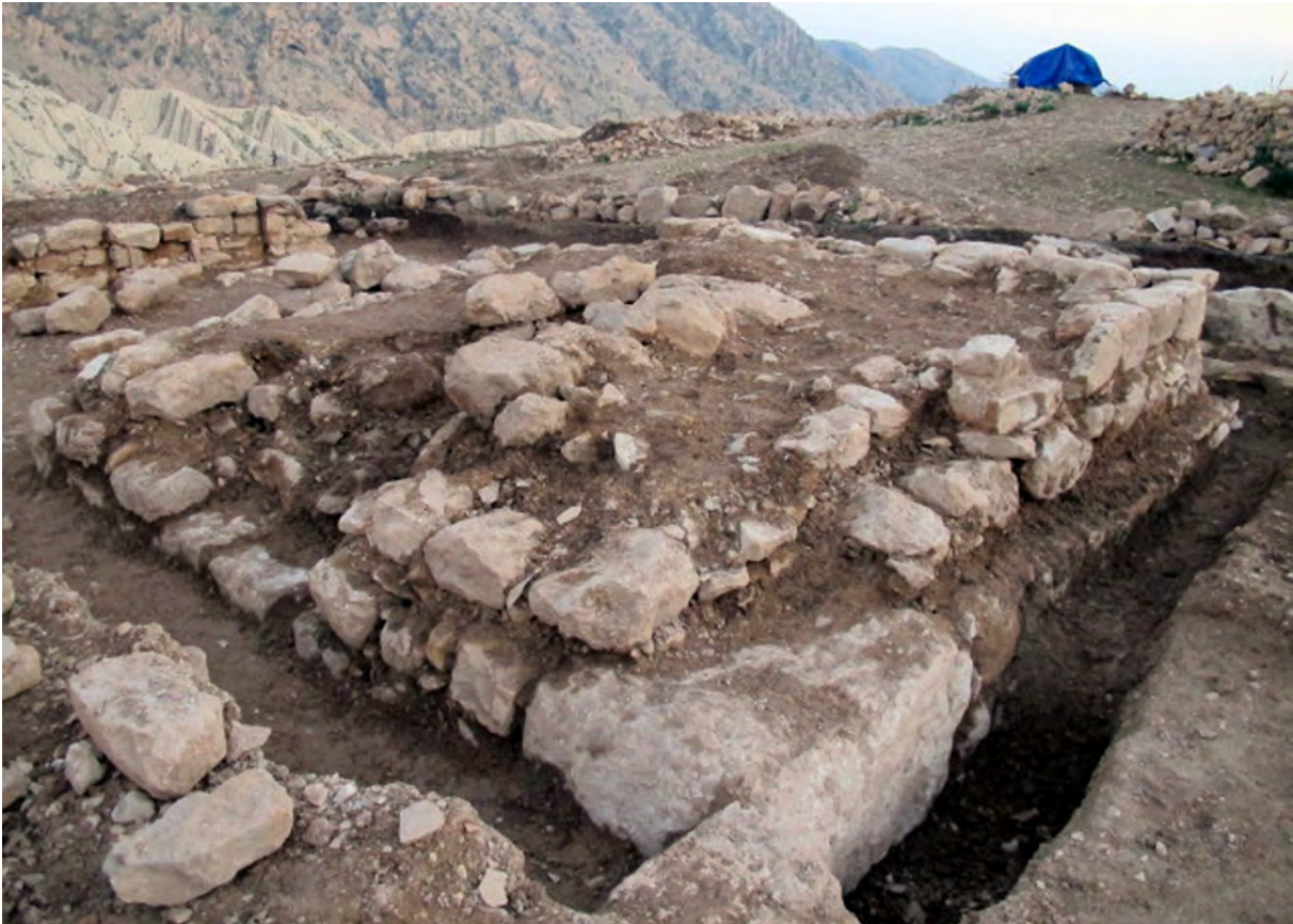
Figure 6.78 - Trench 13. Platform 1 from the northwest
