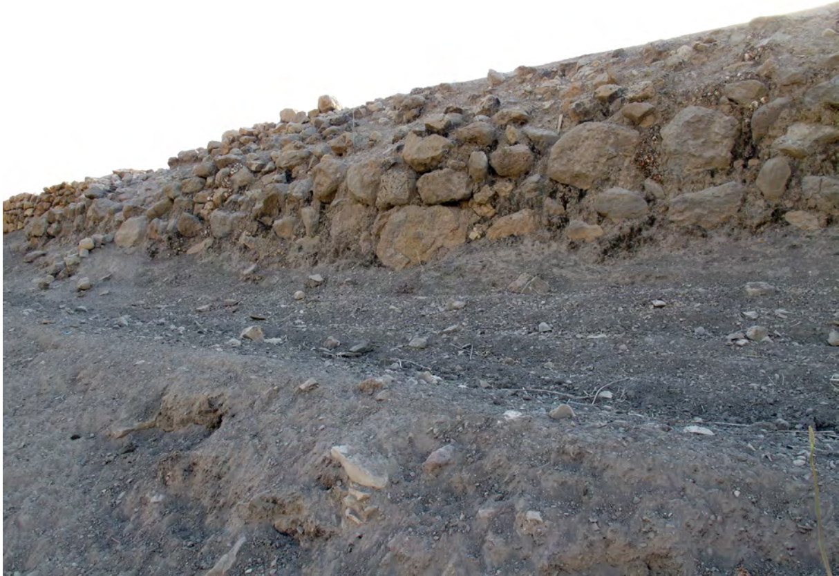
Figure 6.47 - Terrace 3. East retaining wall from the northeast
