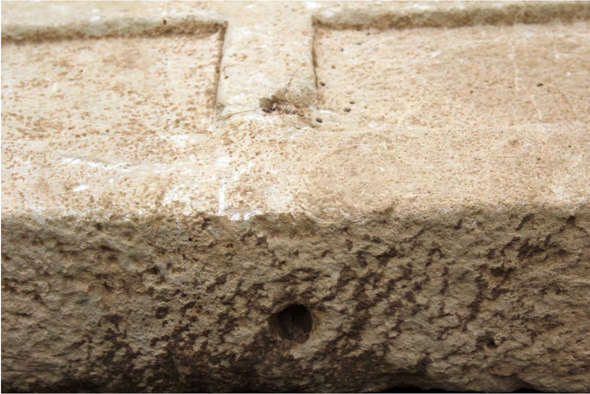
Figure 6.154 - Trench 10. T24. Hinged stone door. Detail of the lock-hole
