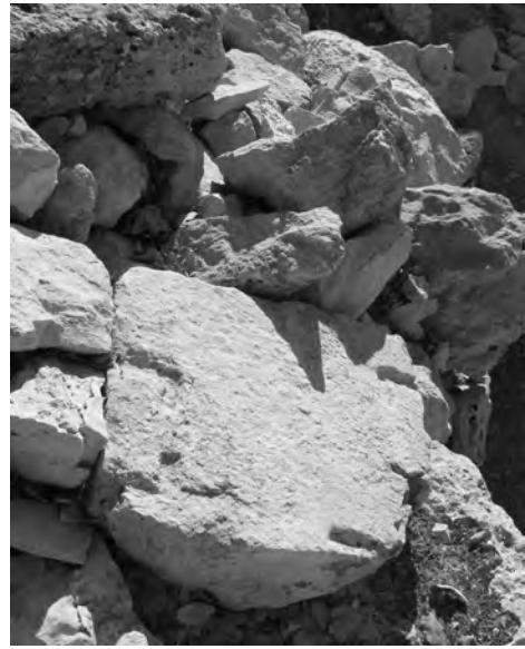
Figure 5.26 - Shami Valley, top of the Bilevah mountain, remains of the qal'eh, detail of the stone masonry with holes for iron clumps
