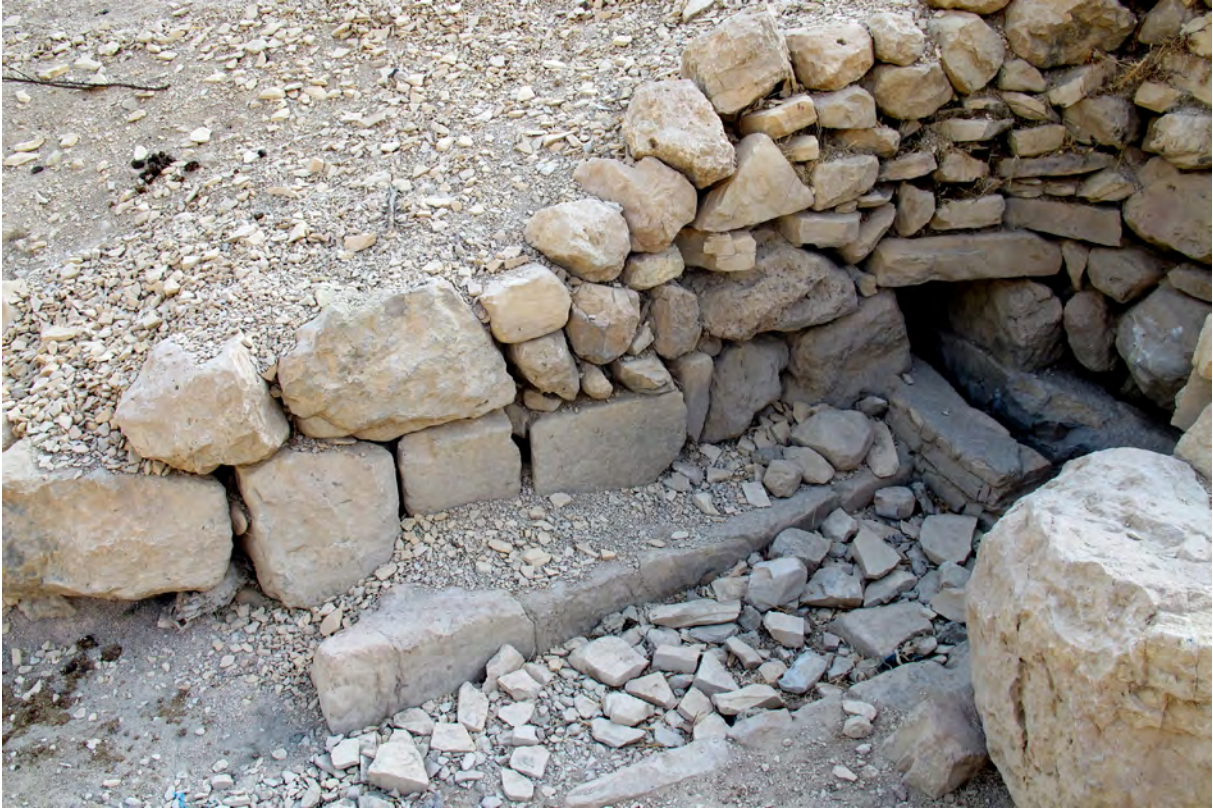
Figure 6.10 - A spring (Spring 1) at the feet of the Upper Terrace's south retaining wall
