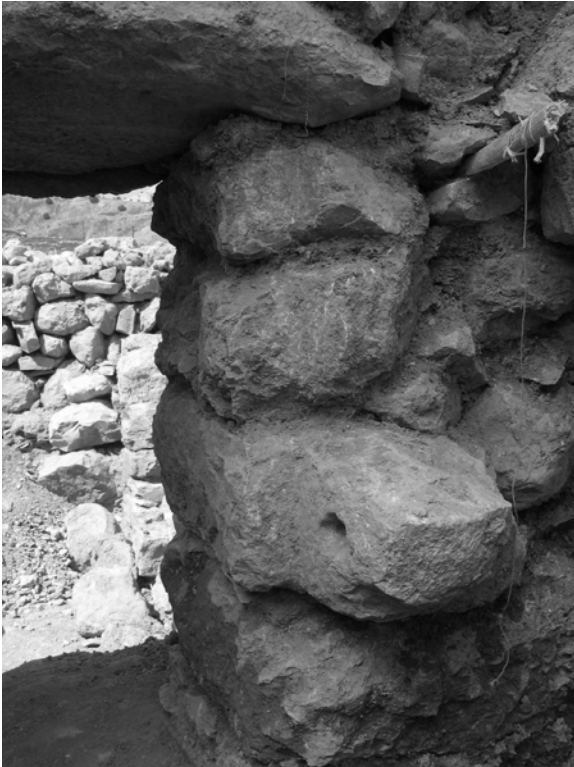
Figure 11.21 - Eastern jamb with a protruding stone with a hole
